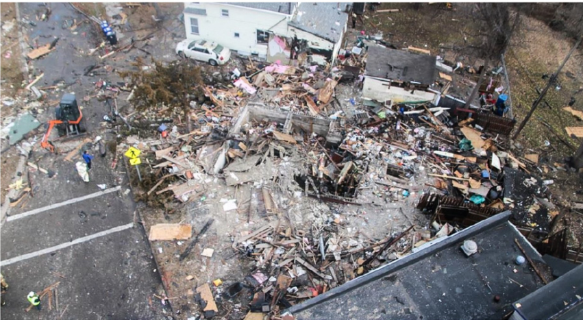
St. Paul fire investigators determined the fatal explosion that destroyed a home on the city's Payne Avenue on Nov. 23 was likely caused by a natural gas leak. The home's owner, John Lundahl, 80, died from injuries sustained in the blast. (Courtesy of the St. Paul Fire Department)
